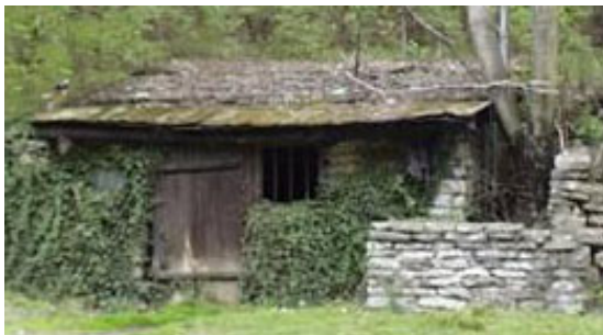
Springhouse Before Restoration
