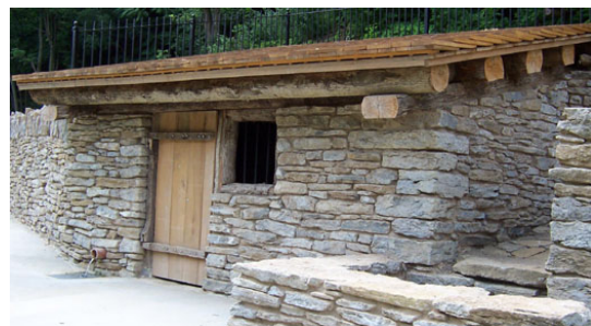
Springhouse After Restoration
