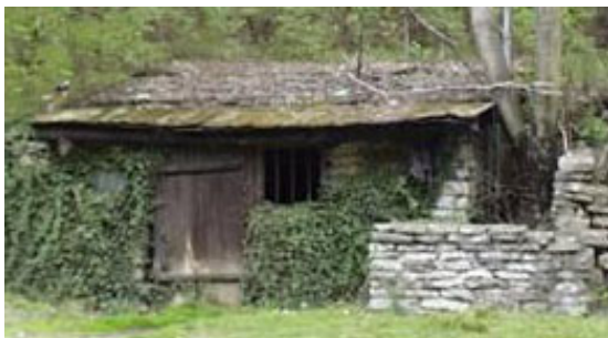
Springhouse Before Restoration
