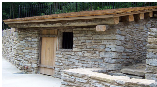
Springhouse After Restoration
