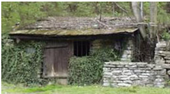
Springhouse Before Restoration
