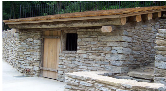
Springhouse After Restoration
